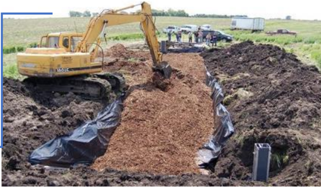
Construction of biofilter
