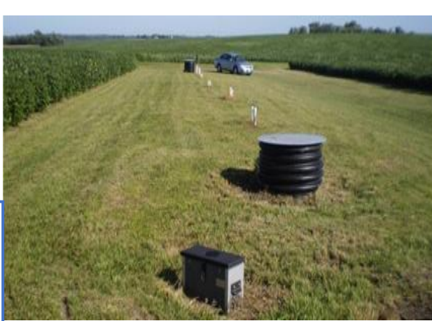
Complete biofilter (6 m x 30 m x 1.3 m)
